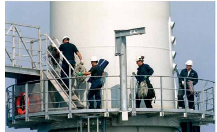
Worker at the tower © Paul Langrock
